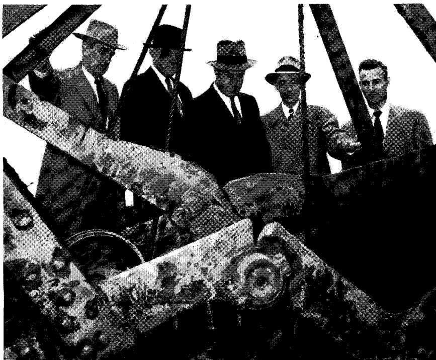
University agronomists and company officials inspect ground breaking for Calumet Nitrogen's new ammonia plant going up at Hammond, Ind. Pictured are: Roger H. Bray, University of Illinois agronomist; E. W. Griscom, vice president, and J. H. Forrester, president, Calumet Nitrogen; Mayor Vernon Anderson of Hammond; and A. R. Bertrand, Purdue University agronomist
